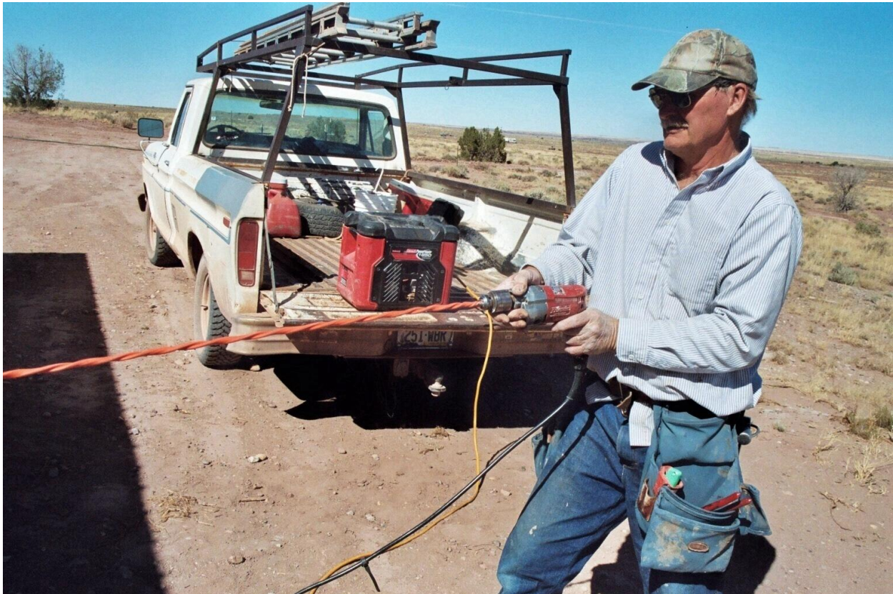
Twisting ROMEX cable, using a power drill
